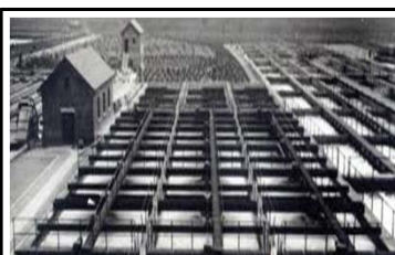
Davyhulme Sewage Works, Manchester, UK, first full-scale activated sludge plant.
